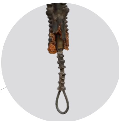
A thick steel-wire cord is threaded through the entire length
